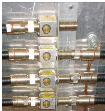
Figure 3 — GDT-based lightning protectors used in the author's station. The GDT cartridge is accessible via the brass screw cap. Each protector is mounted on an aluminum angle bracket that is bolted to the grounded metal sheet.
